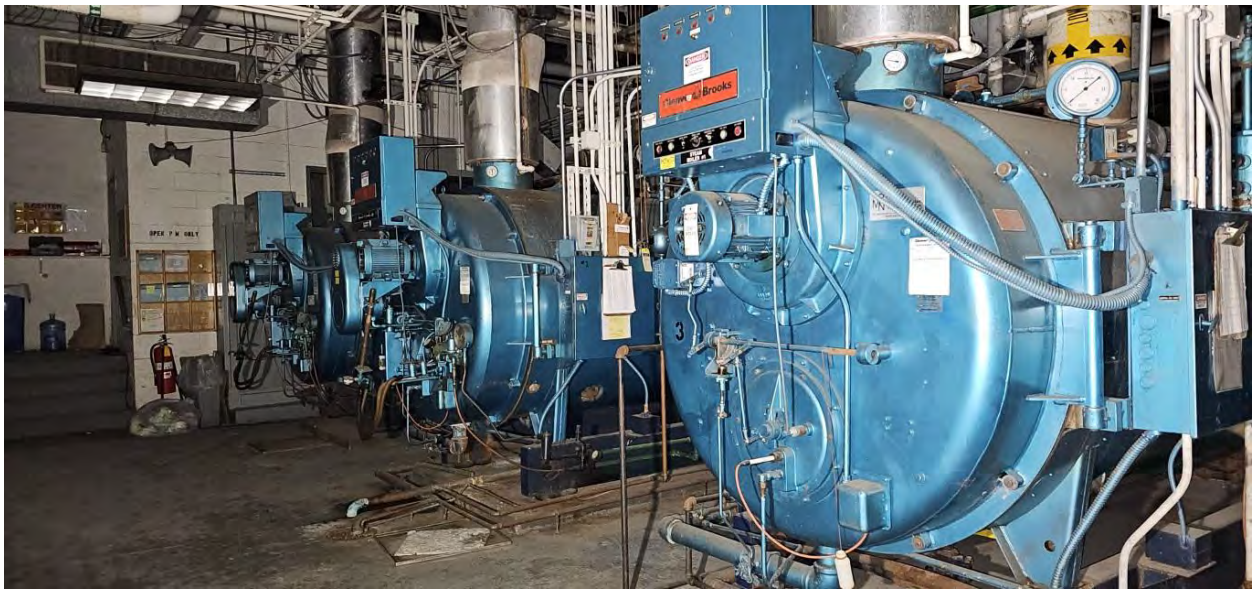
View of oil-fired boiler systems located within the basement of the education building.
