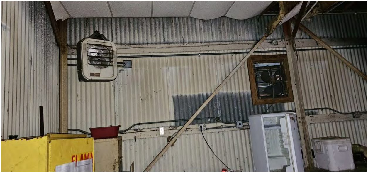
View of an electrical unit heater located within the landscaping/maintenance garage.
