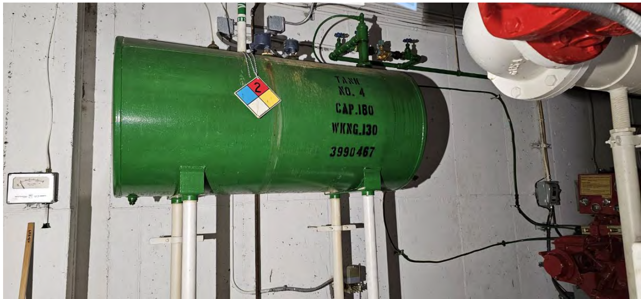
View of an out of service AST located within the basement of the education building which fueled the fire pump.
