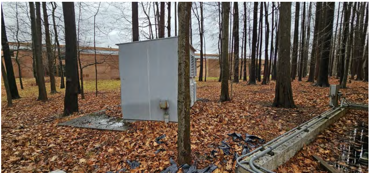
View of a pad-mounted transformer located along the southern exterior of the education building.
