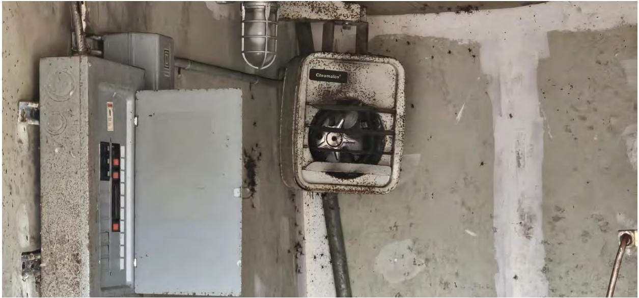
View of an electrical unit heater located within the water shed located along the northwestern portion of the subject property.
