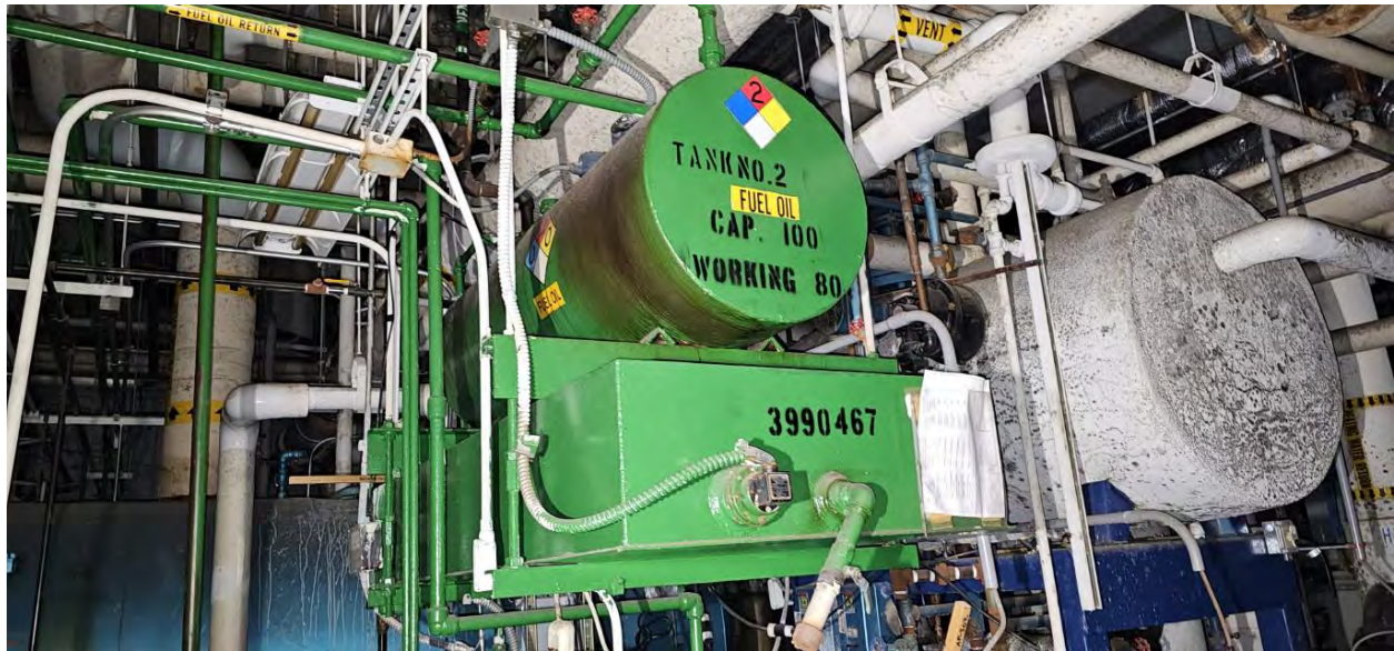
View of an out of service AST located within the basement of the education building which fueled the boiler systems.
